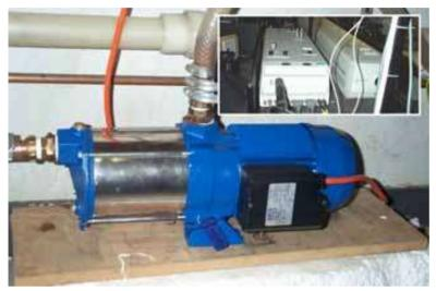
It's a pretty straightforward pump - but its job is extraordinary. Imperial College's Physics Department now boasts an Amos-supplied pump in its Femtosecond Optics Group. Its job is to circulate coolant to an argon-ion laser (that's the larger white box, inset). The laser "optically pumps" the other laser box, which produces femtosecond laser pulses.
